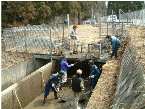
Photo-3: Cleaning water canals
