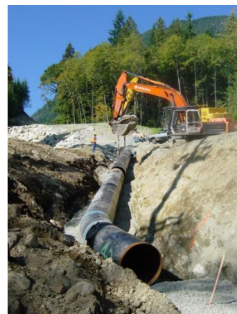
Photo-3 Soil restrained penstock [2]
