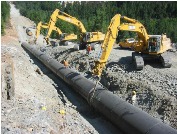
Photo-3. Buried Steel Penstock Construction [2]
