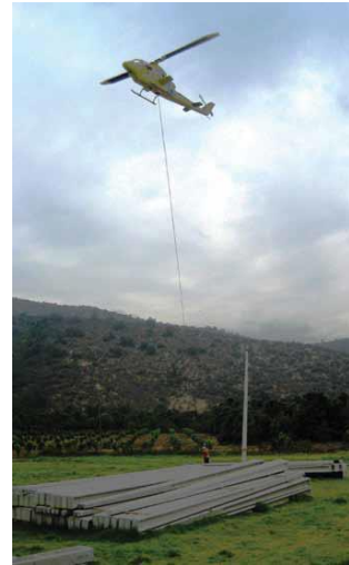
Photo-4 MW line erected by helicopter [2]
