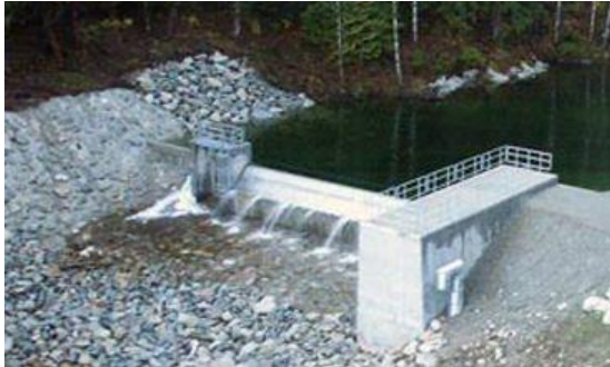
Photo-1 Diversion Weir and Intake [2]
