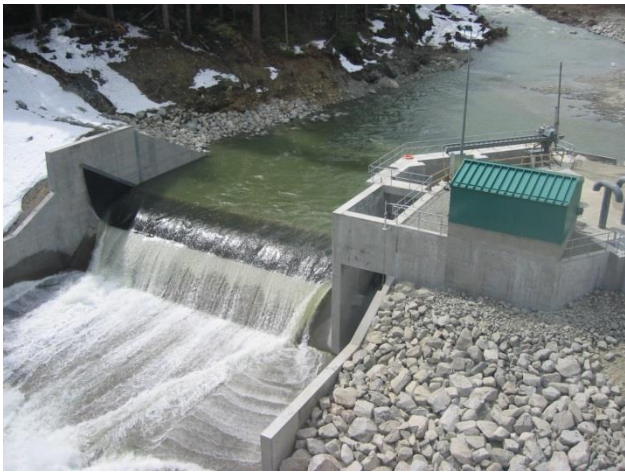
Photo-1 Diversion Weir and Intake [2]
