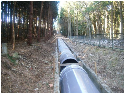
Pipeline (under underground installation)
