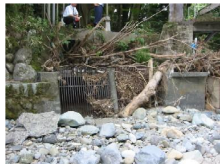
Photo-1: Intake weir and intake (before the renovation)
